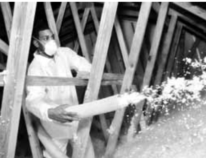
Mark Group installs an energy efficient attic upgrade using EcoFill, a glass-fiber based insulation manufactured with over 60 percent post-consumer recycled material and 100 percent formaldehyde-free. EcoFill is GREENGUARD certified for use in schools and hospitals.
